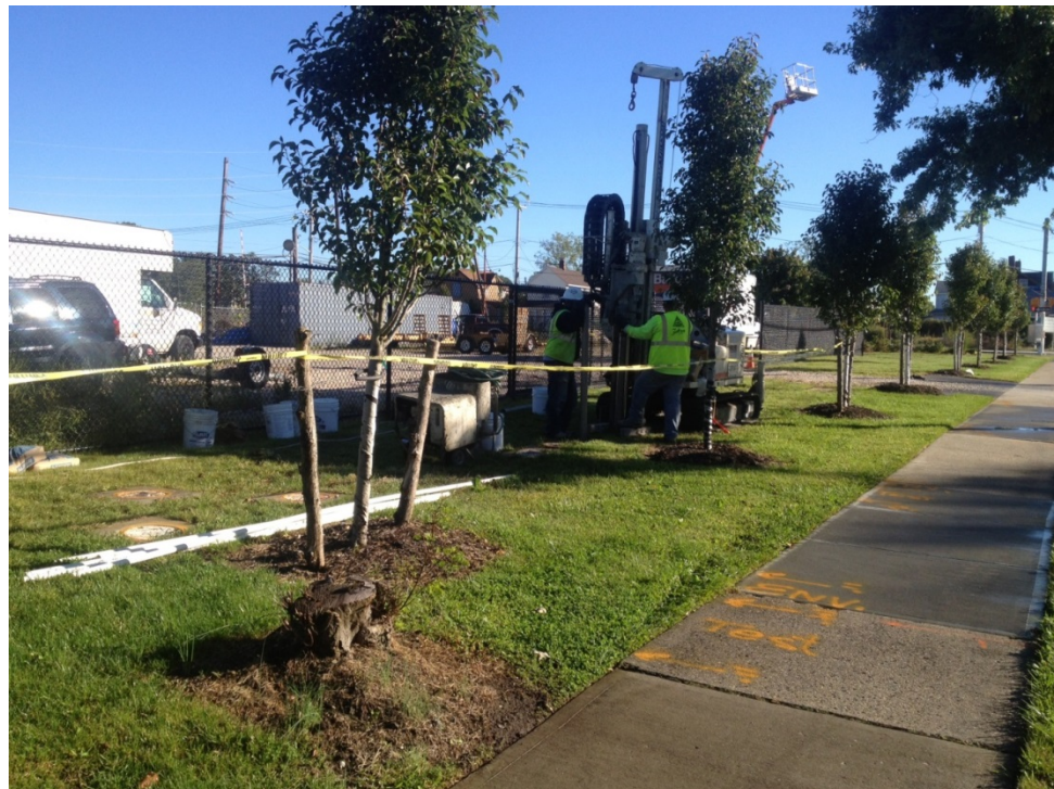
Injection well installation adjacent to Union Boulevard
