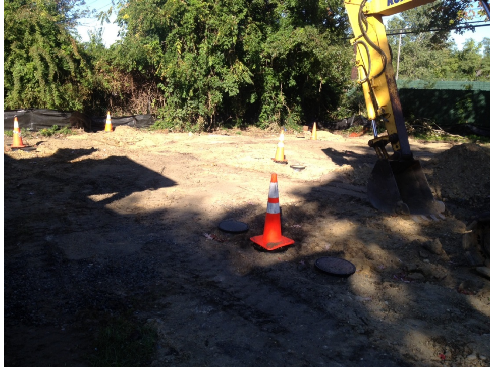
Backfilling and grading at 87 Community Road
